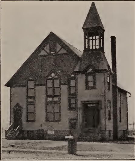
EAST MARKET STREET REFORMED CHURCH, AKRON, OHIO
